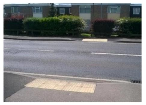
Figure 1 Example of a dropped kerb
