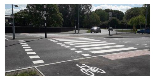
Figure 4- Example of a parallel crossing
