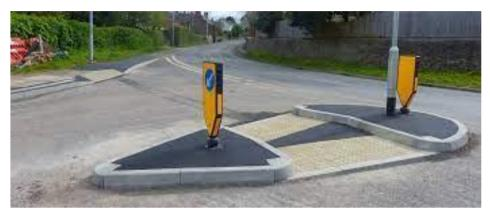
Figure 2 Example of a dropped kerb with a pedestrian refuge
